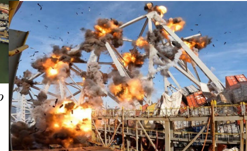
(Below) Explosive cutting of Span 4.
